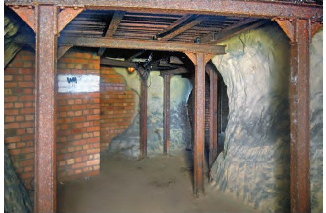
Rouse's is the largest known sand mine in Nottingham, worked from at least 1780 onwards. Together with 75 other former mines in the city it was designated as an air raid shelter in WWII and fitted out with steel strutting and blast walls particularly near its new Peel Street entrance
